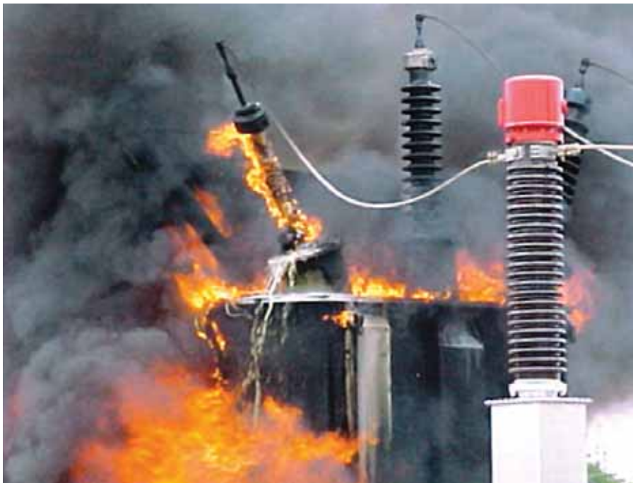
Figure 1: Catastrophic Failure of Bushing
