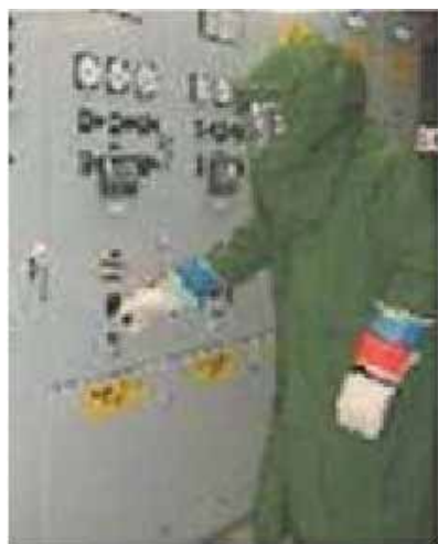
Figure 6: Local switching (Left) vs. Remote switching (Right)
