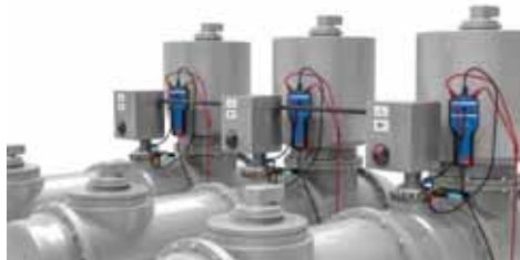
Figure 3: The current sensor is laid around the ground connection of the grounding switch and connected to CB MC2
