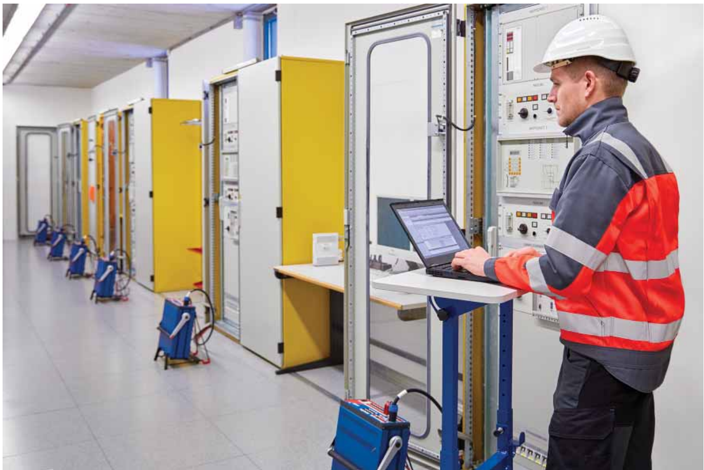
Figure 3: Distributed testing controlled centrally by a PC
