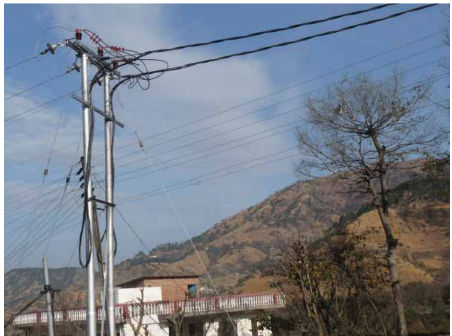
11 KV AB Cable well-installed
