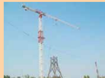
Erection of Tower for Testing
