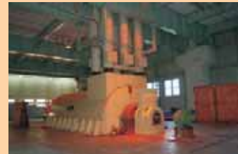
2500MVA Short Circuit Generator
