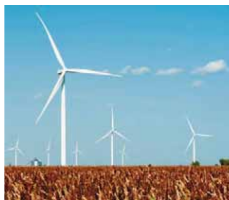
Apex Clean Energy ordered Siemens SWT-2.3-108 turbines for its Kay Wind project...
