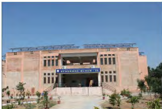
Fig. 1: Academic block ii building, located at "IIT, jodhpur" Jodhpur
