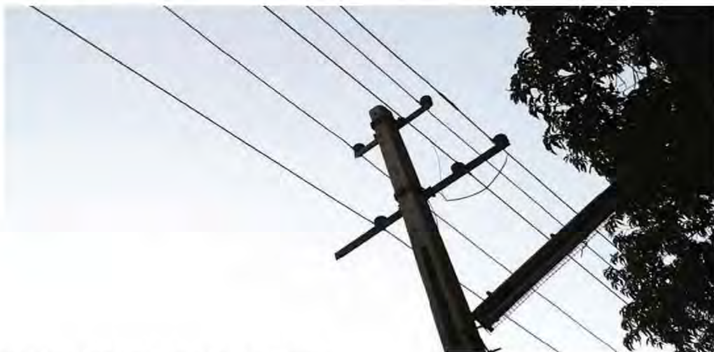
Fig. 5: Present 5 - wire system adopted by the Electric Utilities
