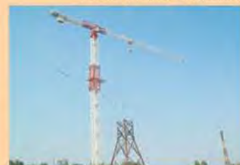
Erection of Tower for Testing
