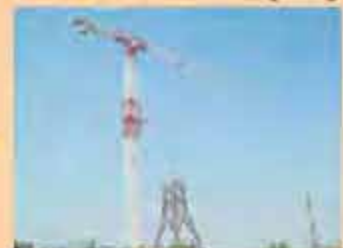
Erection of Tower for Testing
