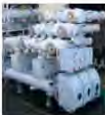
248kV Gas Insulated Switchgear
