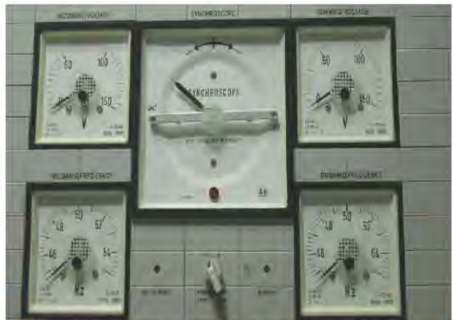
Fig. 1: Synchroscope in a Synch Panel
