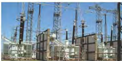
1650MVA, 765kV Class Power Transformers
