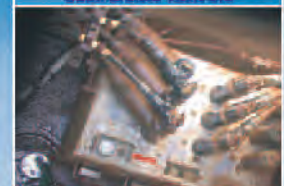
Substation three phase recloser
