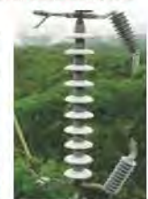
Surge Arrester for Transmission Lines
