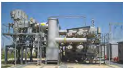
420kV, 63kA Gas Insulated Switchgear
