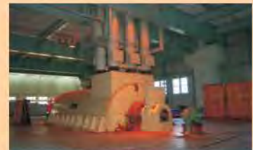
2500MVA Short Circuit Generator
