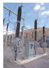
245kV Live Tank Circuit Breakers
