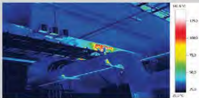
The overheating bearing in a conveyor line is clearly visible.
