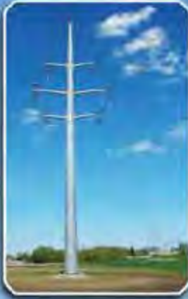
Pole-Type Structure for Transmission Line
