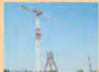
Erection of Tower for Testing
