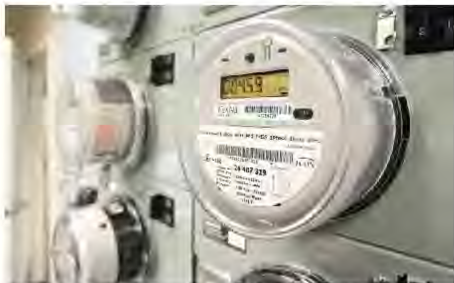
A.B.C. Hydro smart meter, which uses short bursts of radio waves to communication with the electricity grid
