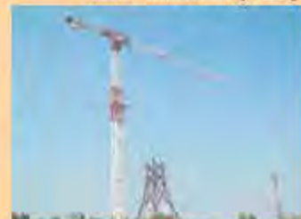
Erection of Tower for Testing
