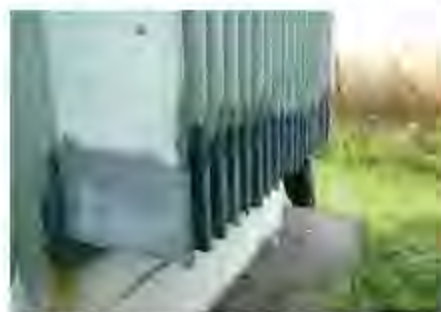
Fig. 9: Oil leakage from radiator...
