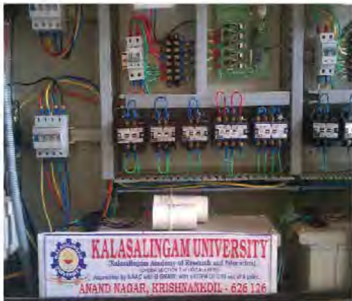
Fig. 17: Photograph of APFC Panel – Kalasalingam University
