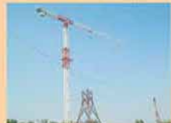
Erection of Tower for Testing
