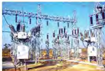
66 kilovolt (kV) and 220 kV hybrid switchgear...
