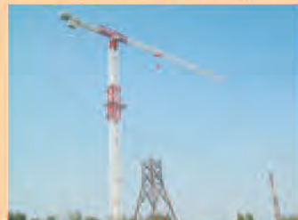
Erection of Tower for Testing
