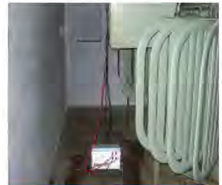
Fig. 6: Winding Resistance Measurement
