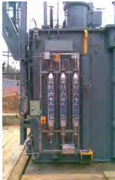
TRANSEC is an on-line molecular sieve, developed and manufactured in the U.K and now manufactured in Facility if Ravin Group under licence from Transec-U.K.
