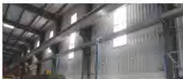
Wide span installation - Supports distance up to 10 meters. Fixed directly in two columns without supports in between.
