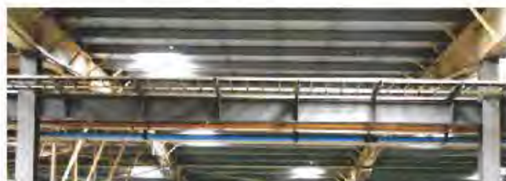
Existing practice - Metallic supports are installed between steel columns and cable trays are fixed in these supports.
