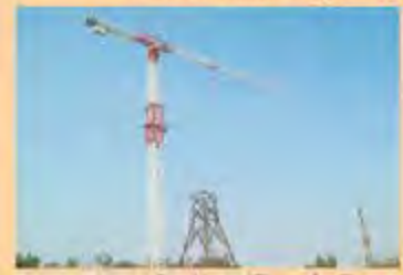
Erection of Tower for Testing
