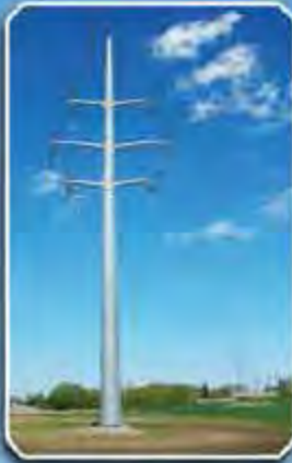
Pole-Type Structure for Transmission Line
