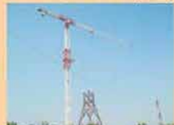
Erection of Tower for Testing
