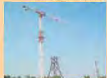
Erection of Tower for Testing
