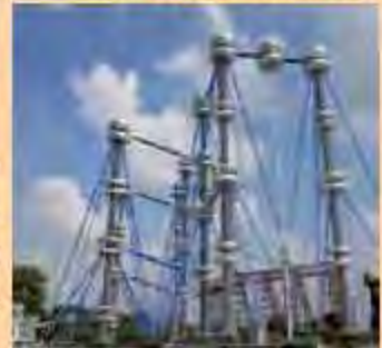
HVDC Generator at UHVRL, Hyderabad
