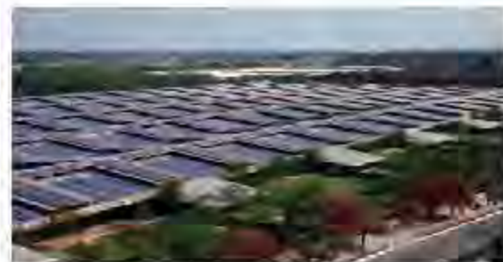
India's largest grid connected solar rooftop plant of 7.52 MW at Dera Beas, Distt. Amritsar, Punjab...
