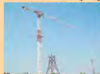
Erection of Tower for Testing
