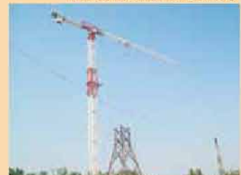
Erection of Tower for Testing
