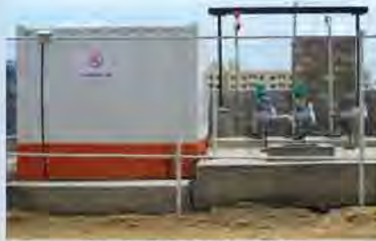
UL Solar Pump testing facility..
