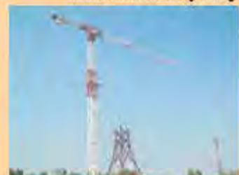
Erection of Tower for Testing
