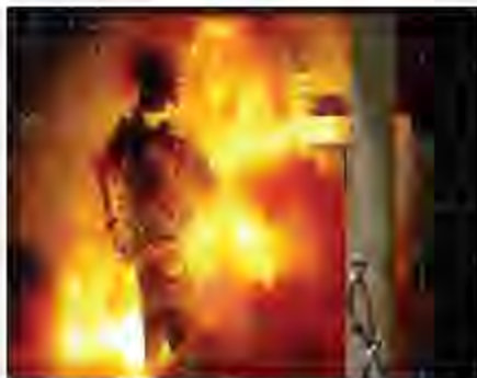
Fig. 1: Arc Flash in a Panel
