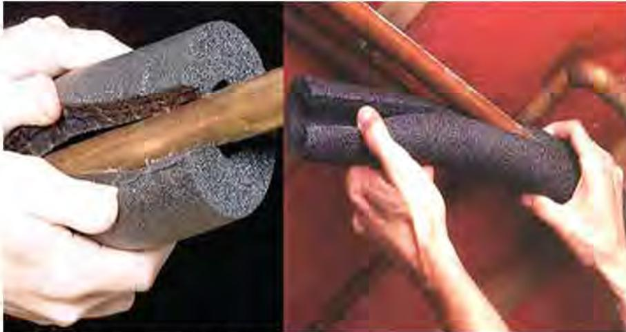
Fig. 3: Heat insulation around hot water pipe line...
