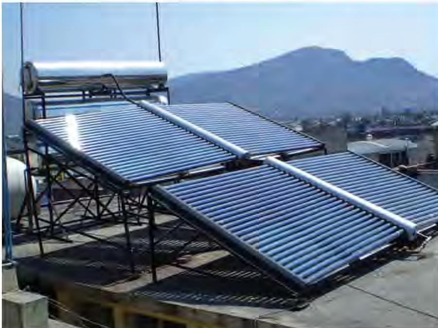
**Fig. 2: 500 LPD solar water heaters...**
