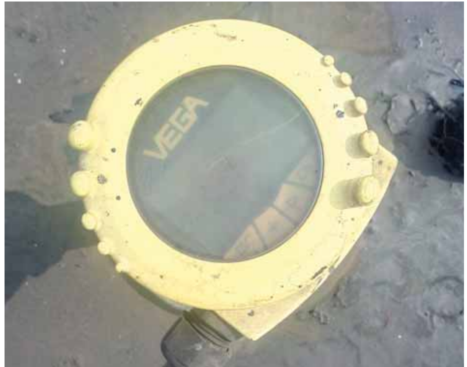
Figure 4: View of level indicator for fuel oil...
