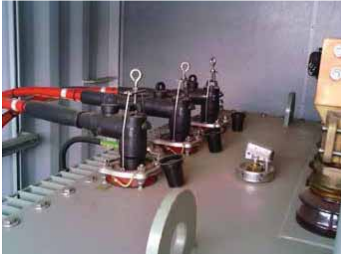
Alternator with abnormality on the primary front plug connector. A bent pin on the angle plug connector is found to be the cause...
