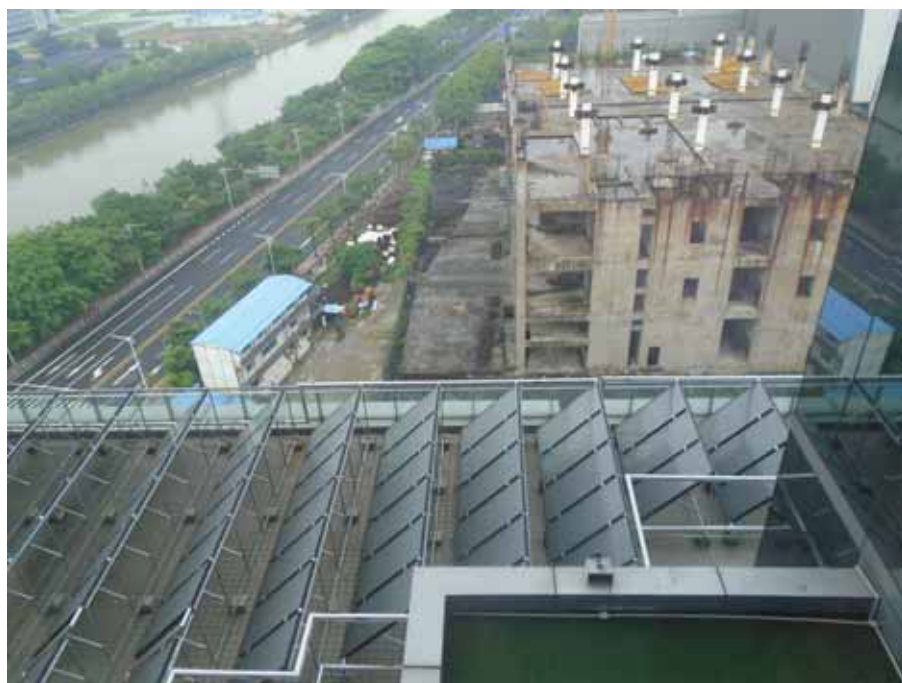
A view of the solar cells installed at Hotel Langham Place, Guangzhou, China...
