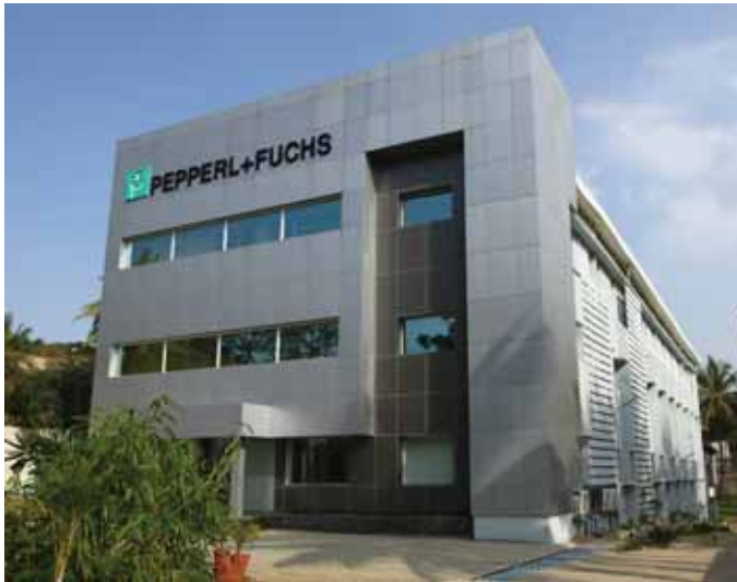
P+F's Indian headquarters and manufacturing unit in Bengaluru...
