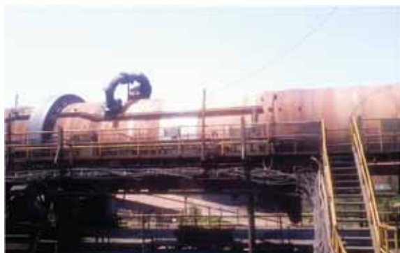
Small white patch: 1st trial of the coating...
