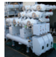
245kV Gas Insulated Switchgear
