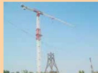
Erection of Tower for Testing
