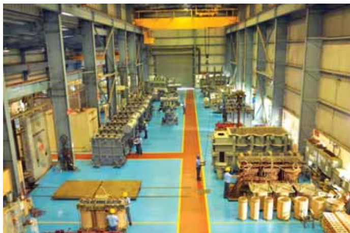
132kV Shop Floor...
