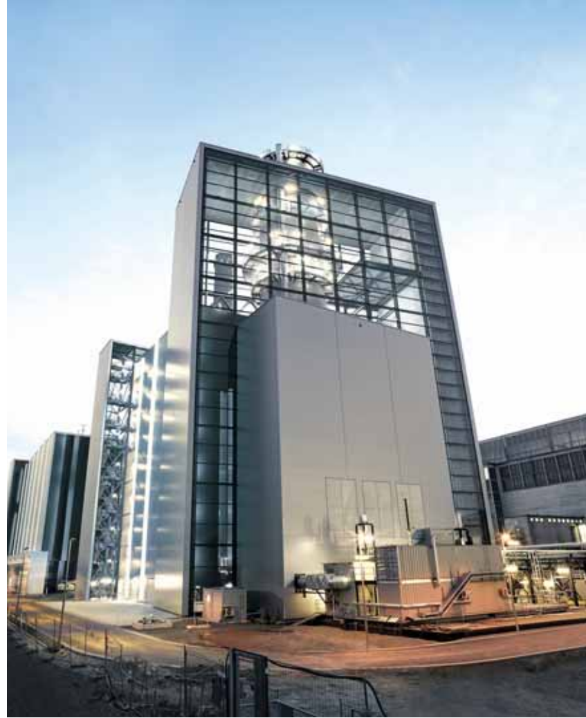
Combined cycle power plant at the location Lausward in Düsseldorf... (Source: Siemens)
