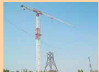
Erection of Tower for Testing
