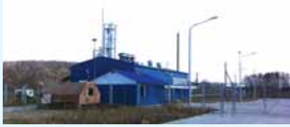
The CHP plant runs on the natural gas producing 1.2 kW of thermal energy per kW of power...
