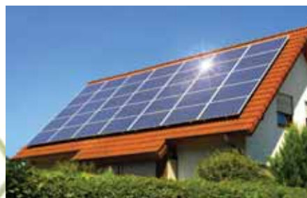
Fig. 3(a): Roof top Solar system...
