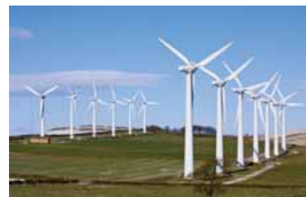
Fig. 3(b): Wind Power Plant...
