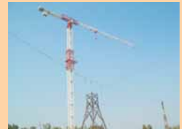
Erection of Tower for Testing
