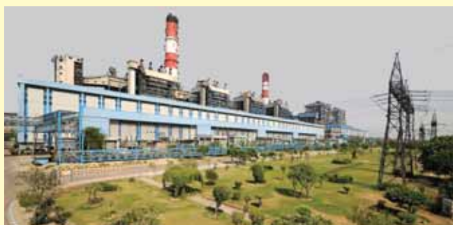
NTPC Dadri, one of the largest power plants in India...
