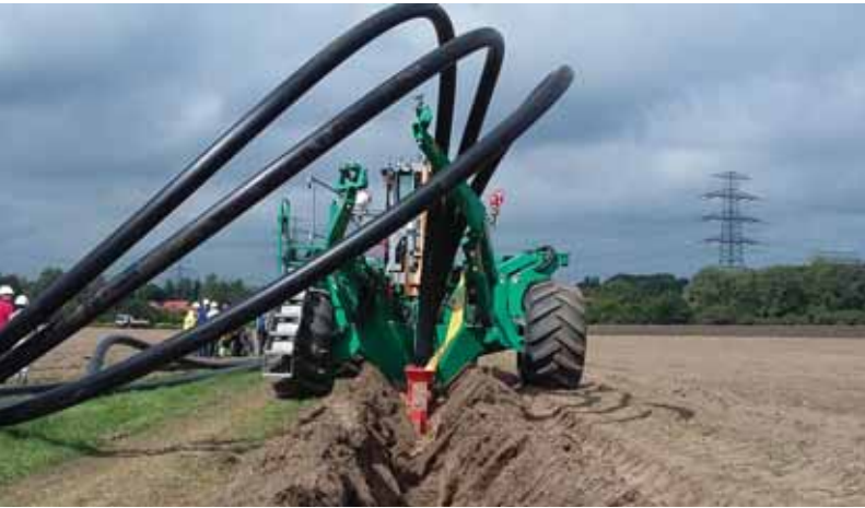
Glimpses from the field where the cable laying work is in progress...
