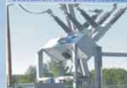
Substation three phase recloser
