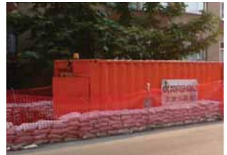
Picture 7: Joint pit cabin made by 20 feet container..
