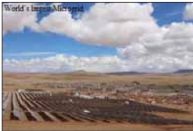
World's largest Microgrid...
