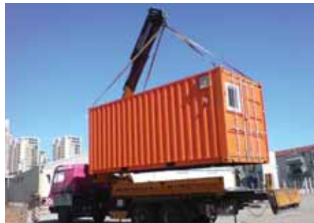
Picture 7: Joint pit cabin made by 20 feet container..
