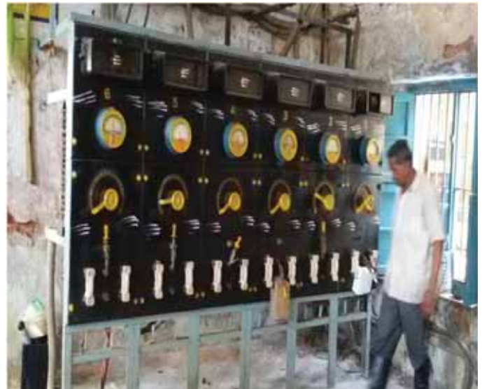
Fig 4: Control panel at railway workshop used for charging and discharging batteries...
