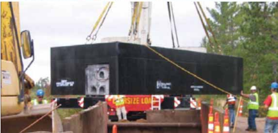
Picture 2: horizontal directional drilling and pre- fabricated joint bay...
