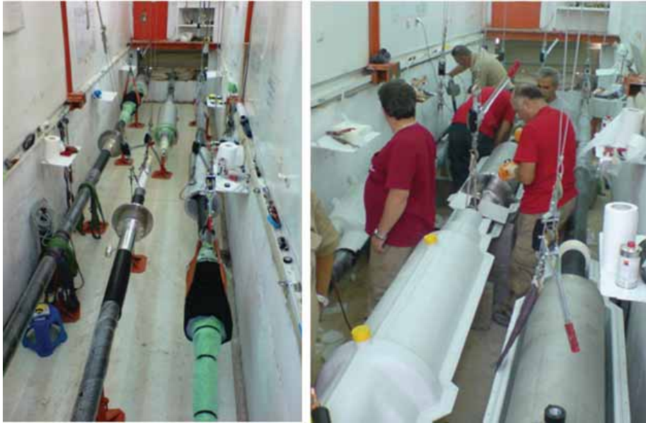
Picture 4: Installation space for joint type MPSP with cylindrical metal casing and horizontal split-box design...
