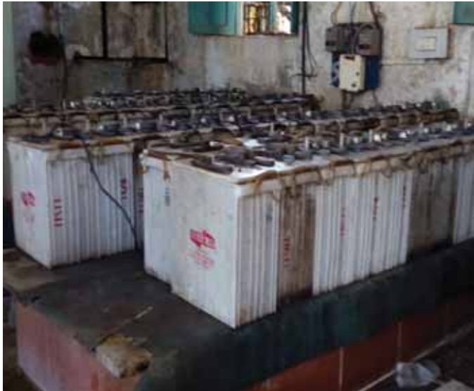
Fig 3: Battery testing in railway workshop...
