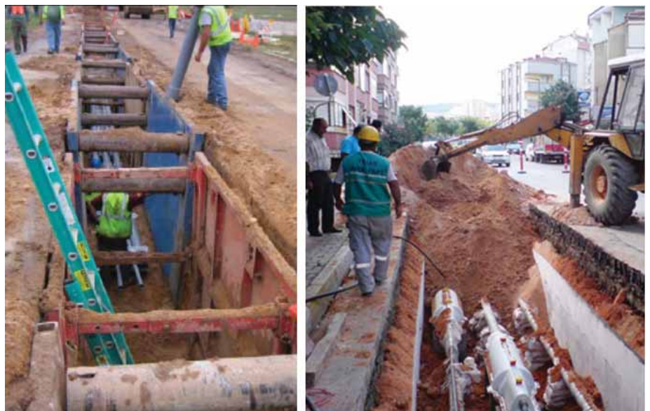
Picture 1: cable and joint installations in open trench...
