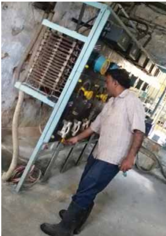
Fig 5: Battery discharging through resistive load...
