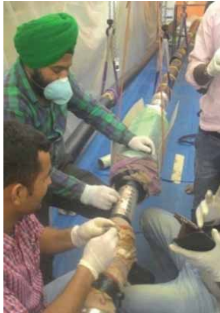
Picture 6: Installation space for joint type MPFP with vertical split-box design...
