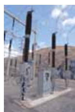
245kV Live Tank Circuit Breakers
