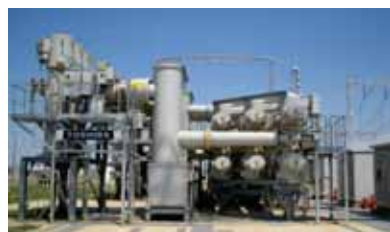
420kV, 63kA Gas Insulated Switchgear
