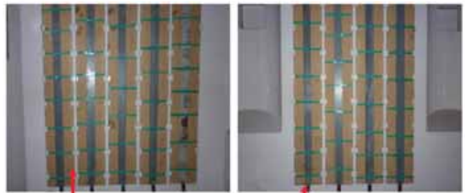
PLACEMENT OF WALL SHIELD & EARTHING ARRANGEMENT
