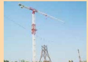
Erection of Tower for Testing
