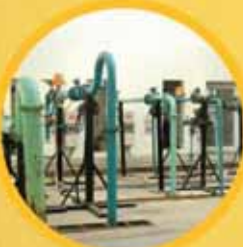
Pump Test Facility
