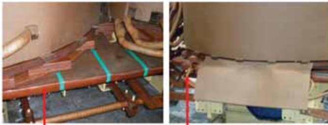
PLACEMENT OF YOKE SHUNT & EARTHING ARRANGEMENT
