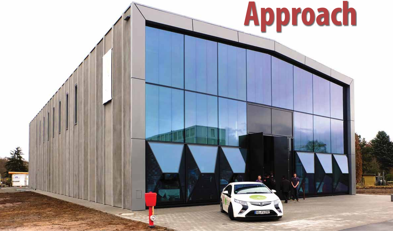
The ETA factory: In addition to improving the energy efficiency of individual production facilities, there the focus is also on linking them in an energy-efficient manner... © Gerhard Hirn, BINE Informationsdienst
