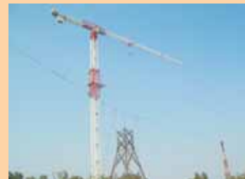
Erection of Tower for Testing
