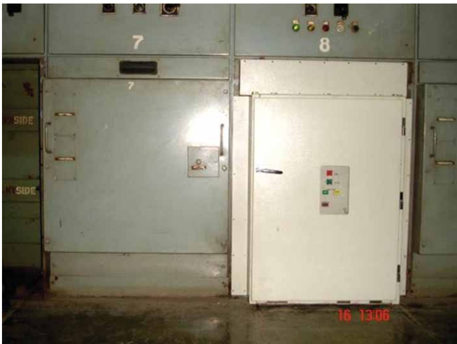
Figure 5: Retrofitted VCB
