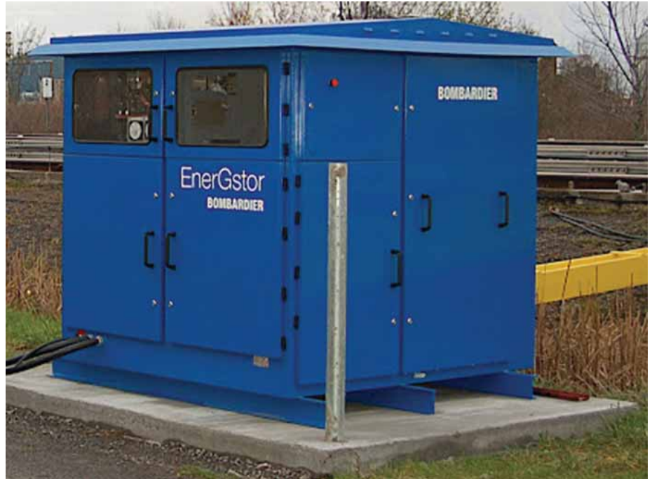
Figure 4: Bombardier's EnerGstor wayside energy storage system uses ultracapacitors to store 2KWH energy
