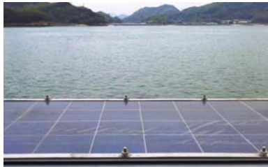
Marine grade solar panel and frame at Teramoto Iron Works, Onomichi, Japan
