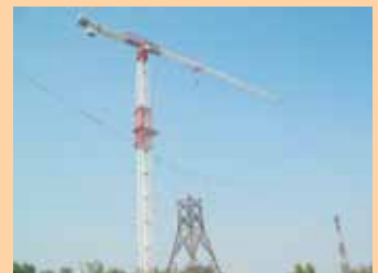
Erection of Tower for Testing
