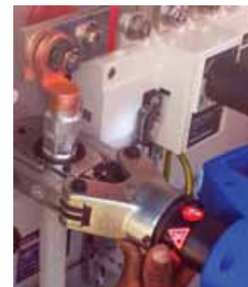
Recently completed project in South Gujarat
