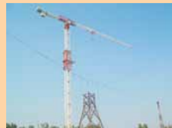
Erection of Tower for Testing
