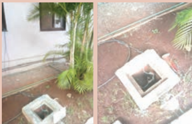
Figure 3: Ground pit with earth electrode
